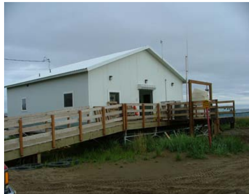
The new Mekoryuk halibut plant
