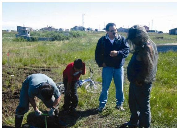
Soil testing at the proposed Eek Fisheries Support Center site
