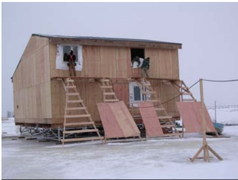
CVRF residents constructing the fisheries support center in Scammon Bay
